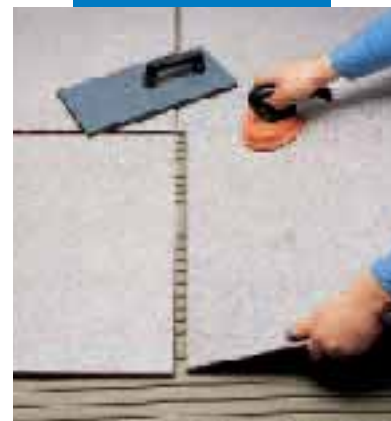
Laying 60x60 cm single-fired tiles
