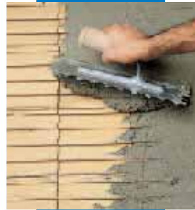
Back-buttering ribbed extruded tiles
