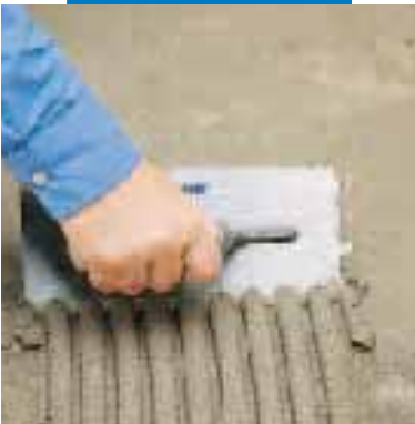
Spreading with the semicircular-notched trowel
