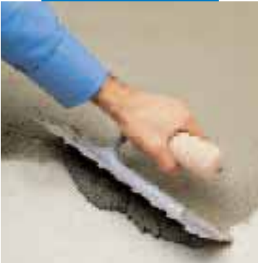
Spreading the preliminary skim-coat
