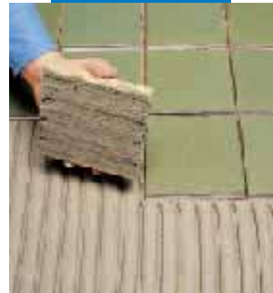
Laying extruded tiles
