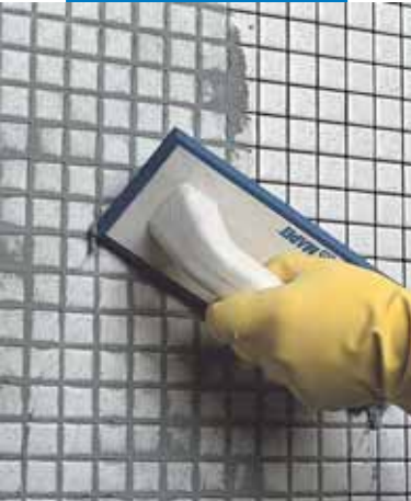
Grouting a glass mosaic (bathroom) with a trowel
