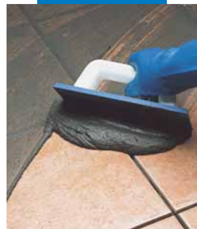
Grouting single-fired tile with a trowel
