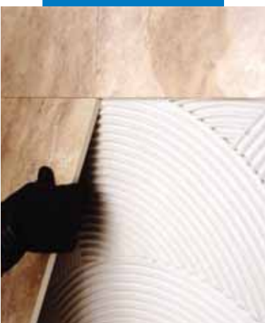
Laying large-sized porcelain tiles on walls
