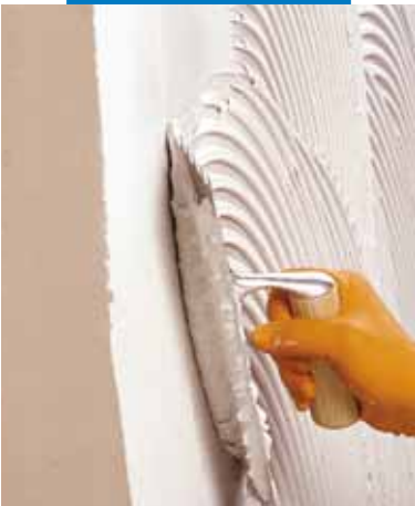
Spreading Tixobond Fine S1 on a substrate
