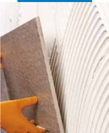
Laying large-sized, double-fired tiles on wall starting at the top and working downwards
