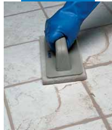
Finishing with a Scotch-Brite® pad
