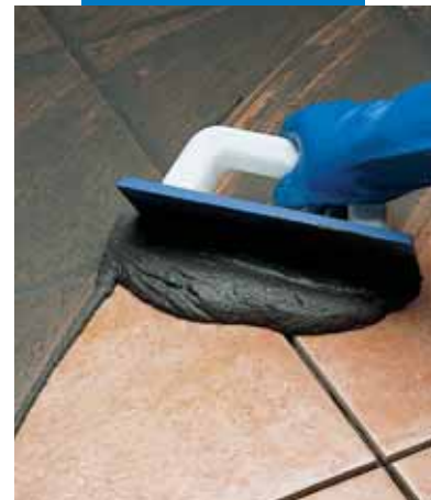
Grouting single-fired tiles with a float
